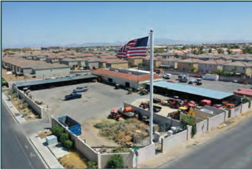
A maintenance facility at Spanish Trails Country Club, Nevada
