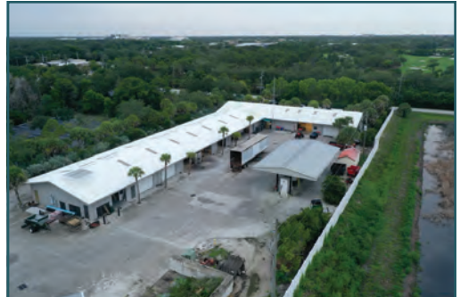
Golf club maintenance facilities
